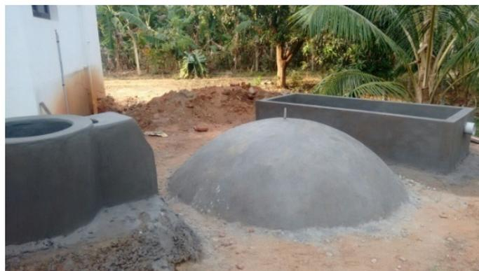
Night Soil cum Kitchen Waste based Biogas Plant is the integration of modern biogas technology with disposal of night soil and food wastes generated from hostel kitchens and dining halls for harnessing bio-based energy.
